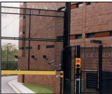
Vertical Lift Gates
